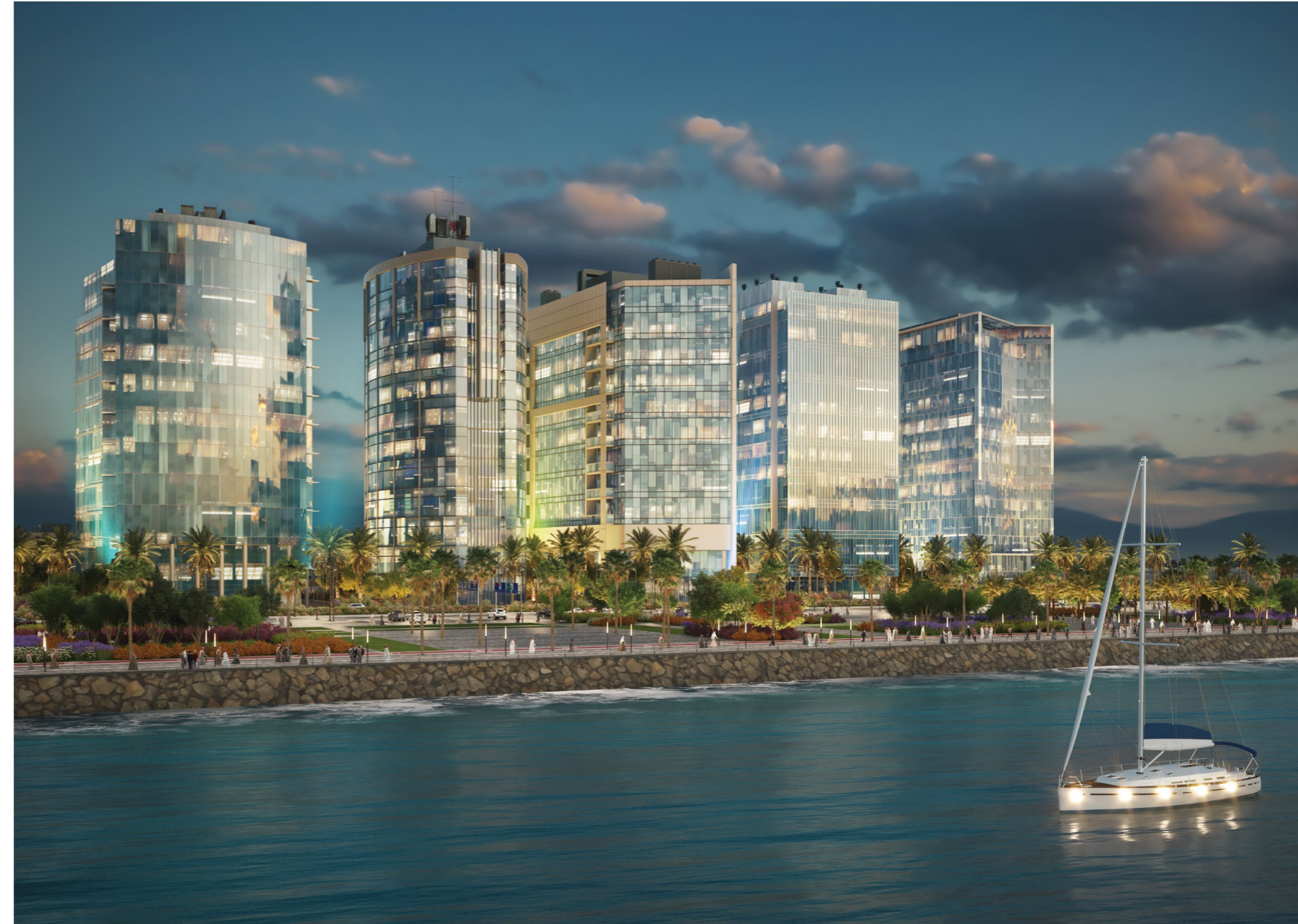
BUSINESS TOWERS 15 FLOORS
