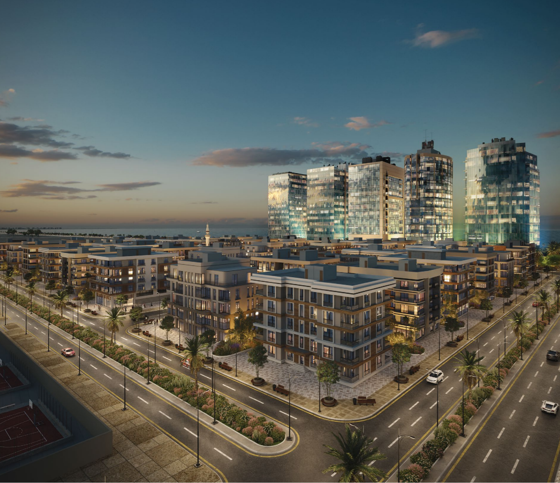
RESIDENTIAL BUILDING 4 FLOORS
